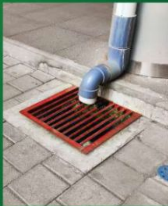
Provision of concealed secondary drain spout to drain accidentally seeped water.
